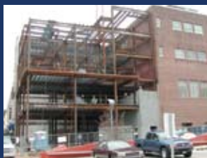
Cosmopolitan Restaurant Under Construction
